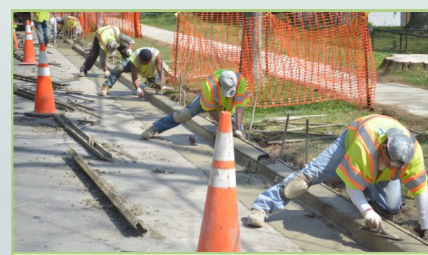
Concrete is smoothed and finished
